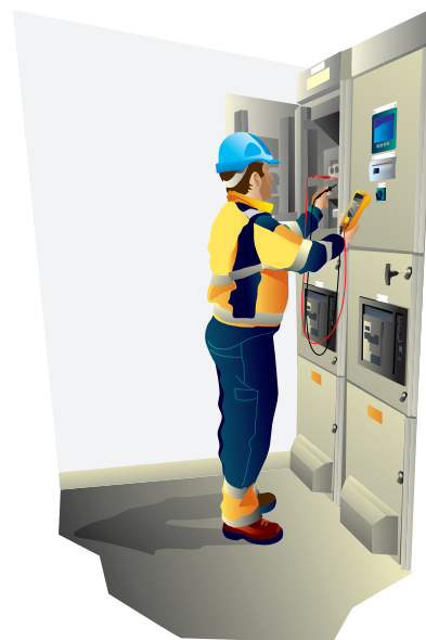
Figure 6. Voltage testing in a low-voltage switchgear.
