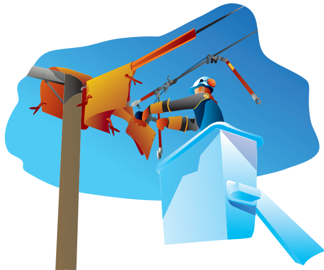
Figure 32. Live working , AMS work with insulating glove.
