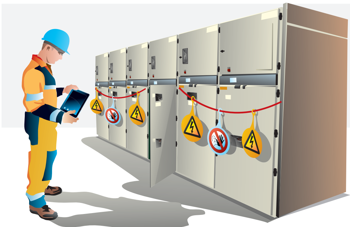
Figure 19. Example of a barrier rope at an indoor switchgear.
